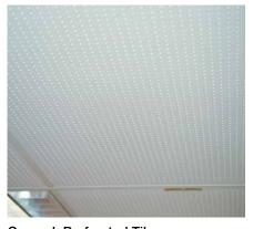
**Gyprock Perforated Tiles** Specifically developed for use in ceilings where additional sound absorption is required. Perforations are approximately 10% of the tile area, and combined with suitable insulation, provide a medium level of acoustic absorption.
