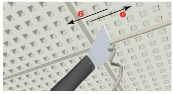
After approximately 24 hours, the joints and covered screw heads can be sanded and prepared for painting. Heavy sanding should be avoided as it may result in surface damage.
