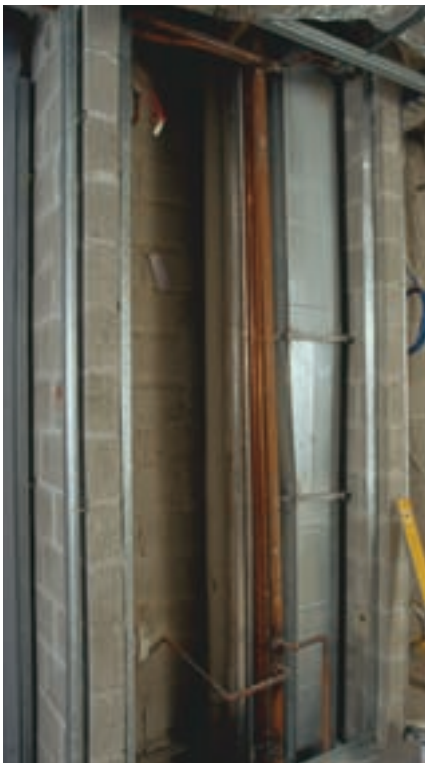
SERVICE SHAFT WITH PERIMETER ANGLE FRAME FIXED
