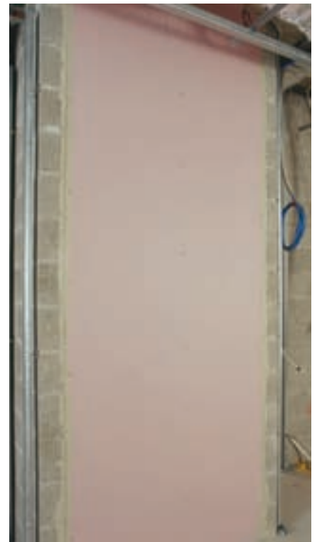
GYPROCK LAMINATED SERVICE SYSTEM AFTER COMPLETION
