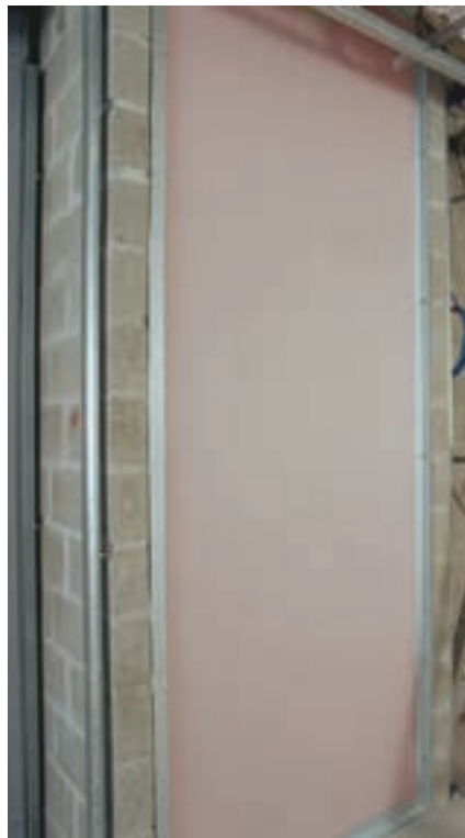
FIRST LAYER OF GYROCK FYRCHEK AND PERIMETER FRAMING FIXED
