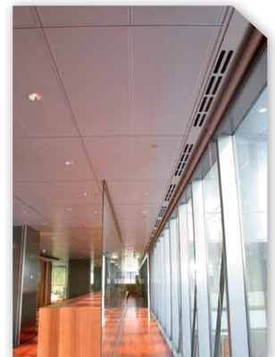
The System 205 Fully Concealed Metal Pan Ceiling at Westpac House, Sydney
