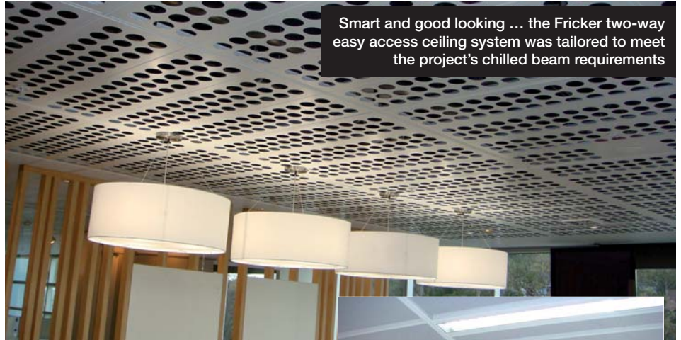
Up in the air ... the perforated tiles allow the correct flow of air through the ceiling system to interact with the chilled beams →
