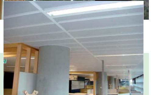
Up in the air ... the perforated tiles allow the correct flow of air through the ceiling system to interact with the chilled beams →
