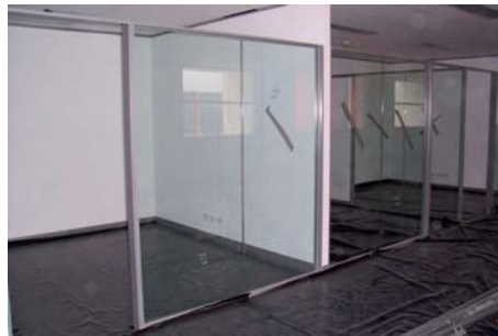
The office and warehouse space was fitted with 1,500m 2 of EC08
