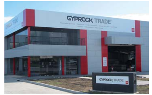
In service ... the new Bayswater Gyprock Trade™ centre
