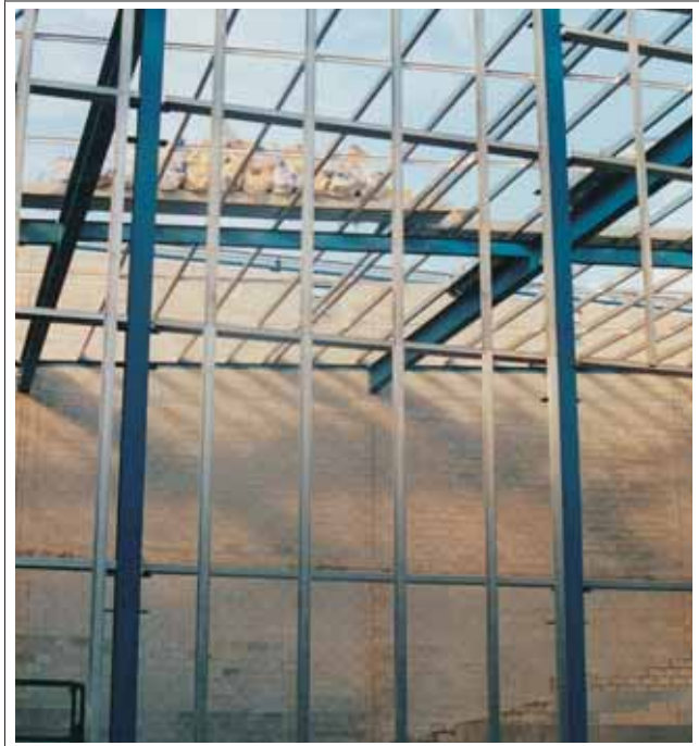
CINEMA WALL DURING CONSTRUCTION.
